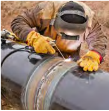
Figure 12. Manual Metal Arc Welding.
