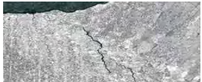
Figure 7. Typical hydrogen induced cold crack in a T-fillet weld.
